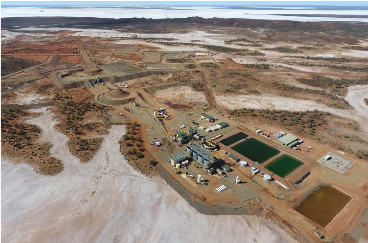
Figure 3: Corresponding photograph to Figure 2, showing the completed 2.5Mtpa treatment plant. This photograph was taken exactly 10 months after the photo shown in Figure 2, on the 24 th March 2018.
