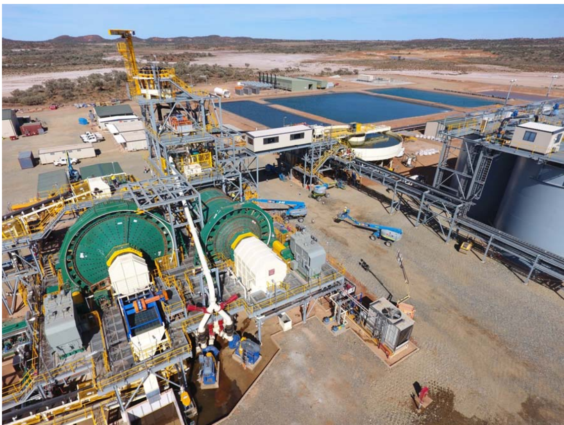
Figure 5: SAG mill and ball mill assembly with CIL tanks of the new 2.5Mtpa treatment plant at Mt Morgans. Note the treatment plant ponds and power station behind the mills and tanks. See also Figure 3 for reference.
