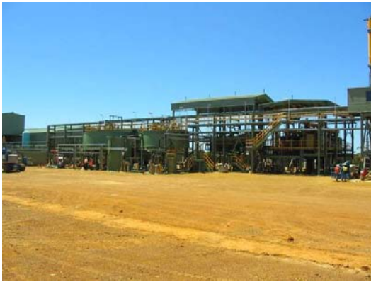
Fig 4. Flotation and concentrate and tailings thickeners
