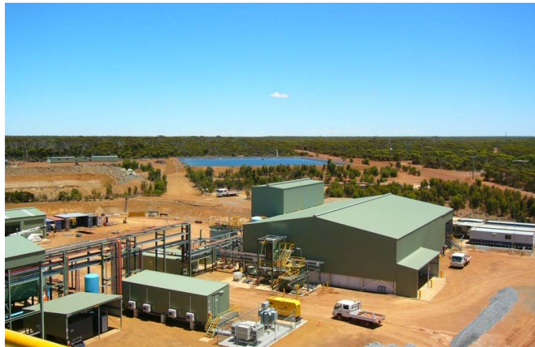
Figure 6. View from Coarse Ore Bin looking west. LHS Cosmic Boy Decline; centre Filter and Concentrate Storage Shed; rear Process Water Storage
