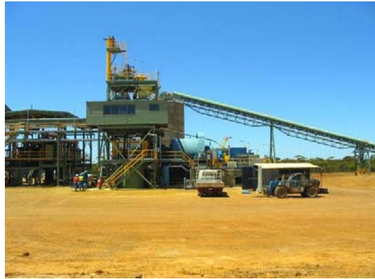
Fig 5. Grinding circuit and control room
