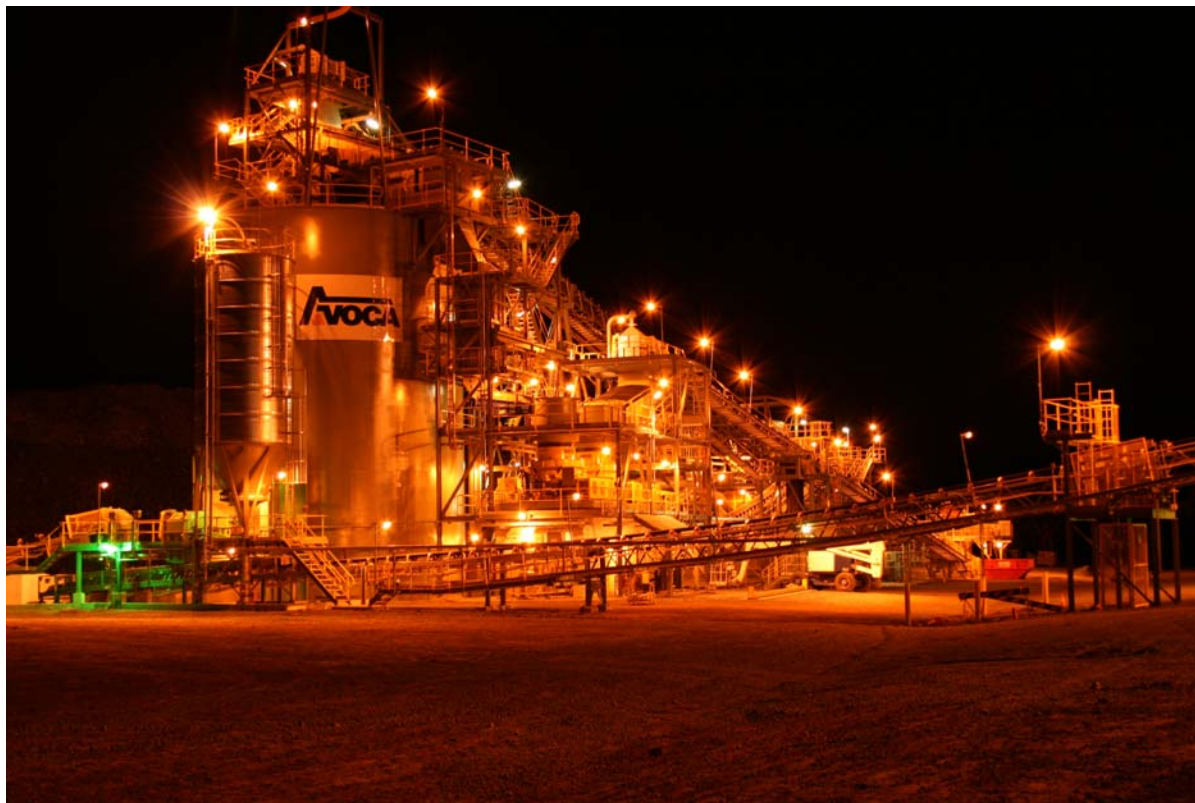
Figure 1: Avoca's Higginsville Treatment Plant has been completed on time and within budget.
