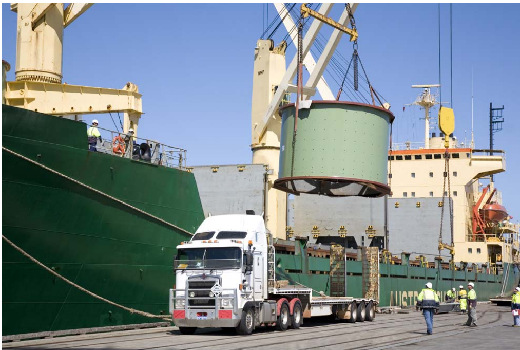
Figure 1: One of the two ball mill shells being unloaded from a cargo ship prior to its delivery to site.
