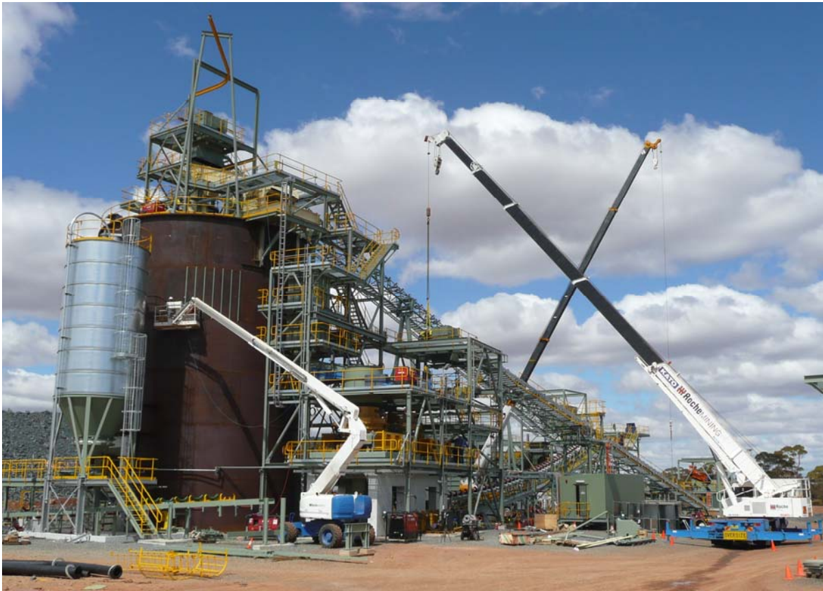
Figure 2: Crushers and fine ore bin assembly at the Higginsville treatment plant.
