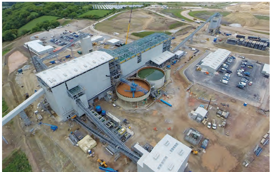
Britain's first new metals mine in over 40 years, Hemerdon, was brought online this year. GR designed, constructed and commissioned the 3 mtpa tungsten and tin processing plant
